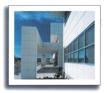
Thinshell wall panels use less concrete than other concrete wall systems. Less concrete equals less weight and greater efficiency.
