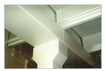
Precast, prestressed beams and columns are plant fabricated building components used to support other elements of a structural system. They are an integral part of any complete precast system, but can also be used easily with any combination of materials.
