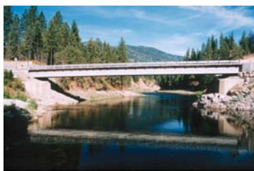
Bulb Tee , 56' to 90' spans.
